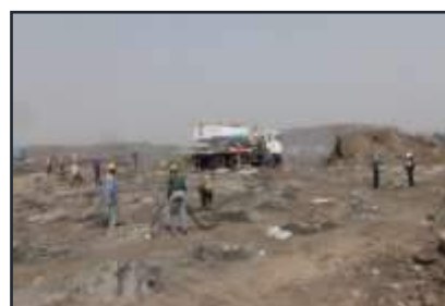
Figure 3. Charging of holes with SME explosives
