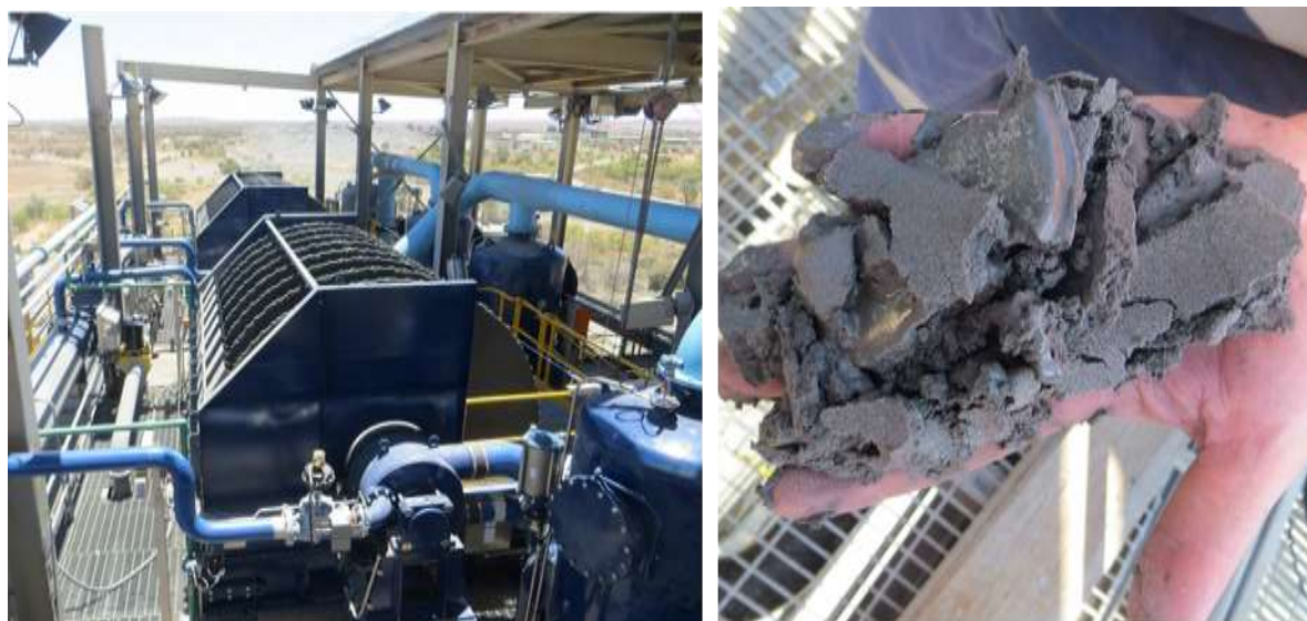
Figure 4. Two Boozer disc filter ME8 (141 m 2 filter area each) for zinc tailings dewatering in the filter building (left); discharged filter cake (right)
