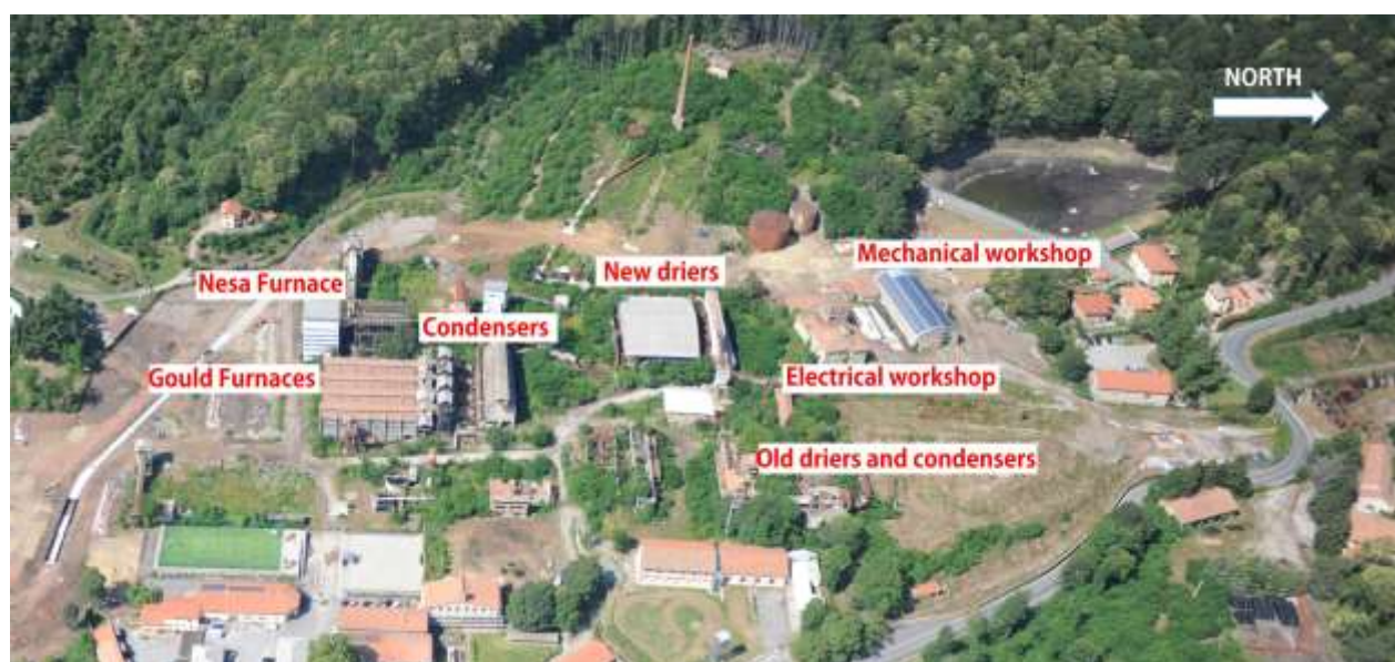
Figure 2. Aerial view of the main edifices and mining structures in the former mining area of Abbadia San Salvatore.
