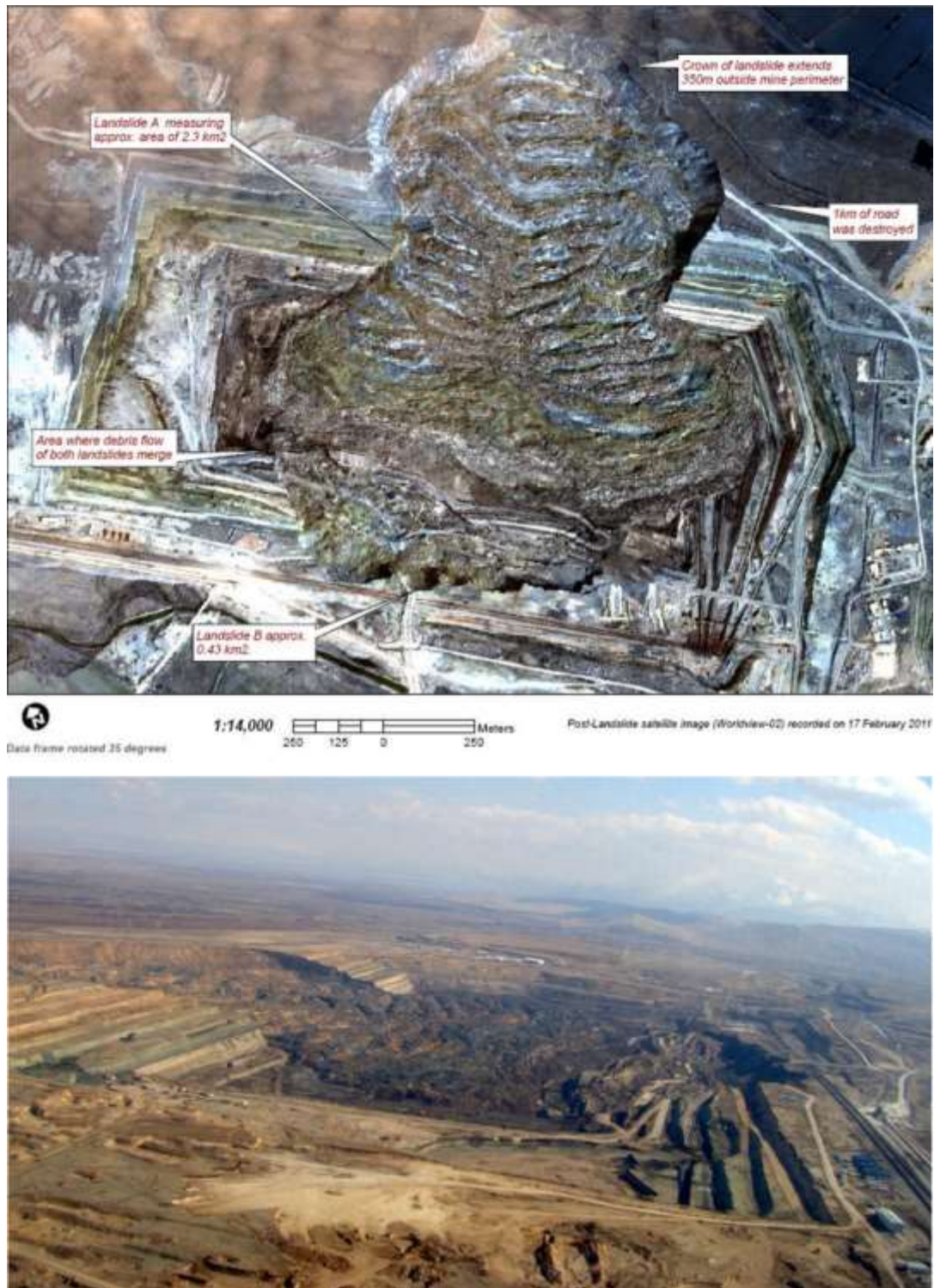
Figure 6. Picture of the slope movement ( http://blogs.agu.org/landslideblog/2011/03/09/the-astonishing-collolar-coalfield-landslide-in-turkey/ ).
